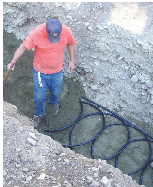
Figure 3 Slinky loop installation.
