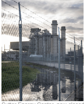
Sutter Energy Center, now closed, made money only if Calpine Corp. found customers for the plant's power. Other large, natural gas plants in the state also face early closures. (David Butow / For The Times)
