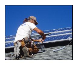
At left, Feather River Solar's Bill Battagin works on the installation of my DC combiner box that heads for the DC-AC inverters, right.
